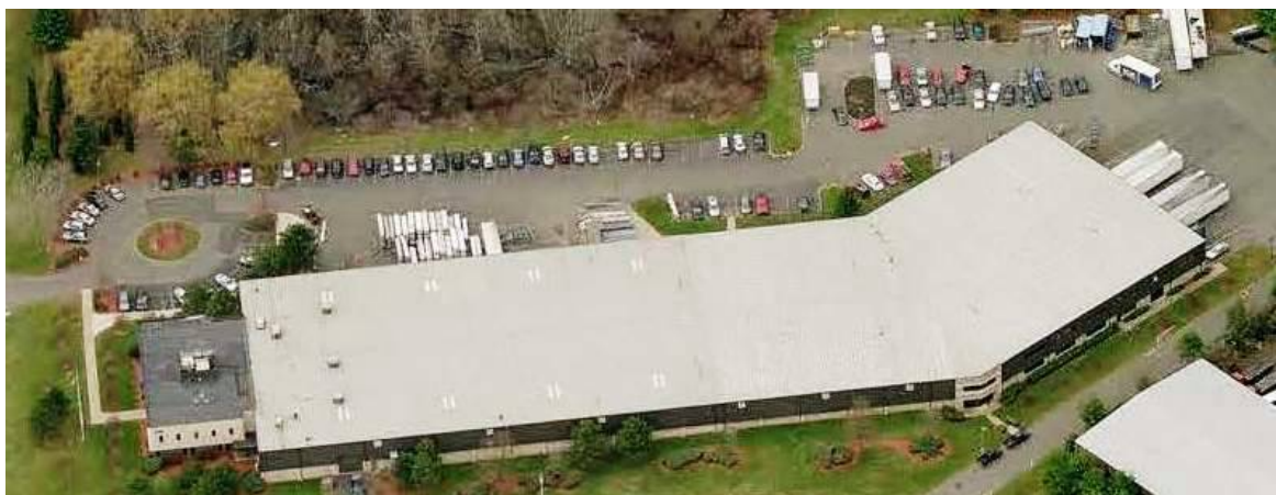
240 Pane Road – Newington, CT
